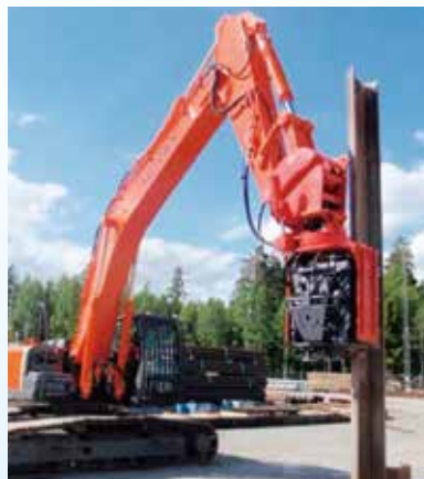
Pitching of pile & Pile installation
