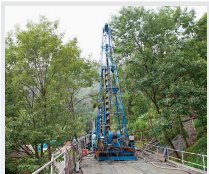
φ550(Landslide control steel pipe piles) L=17.0M~22.0Mx37 Table machine(RTP-680A)
