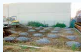
Construction site after complete construction
