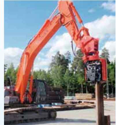
Final pile installation
